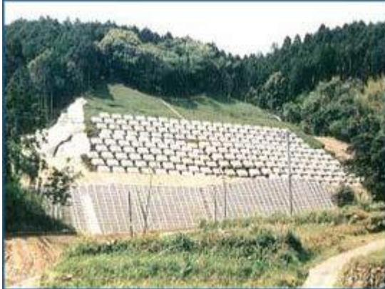
Concrete 'anchors' on a hillside in Japan to help prevent landslides.
