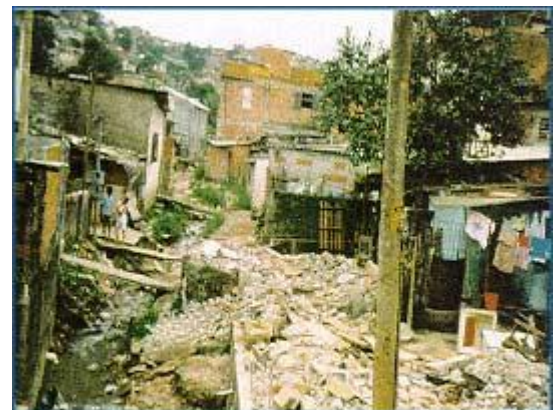
Before slum upgradation
