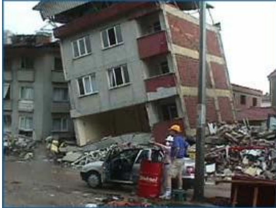
Earthquake liquifaction damage to apartment.
