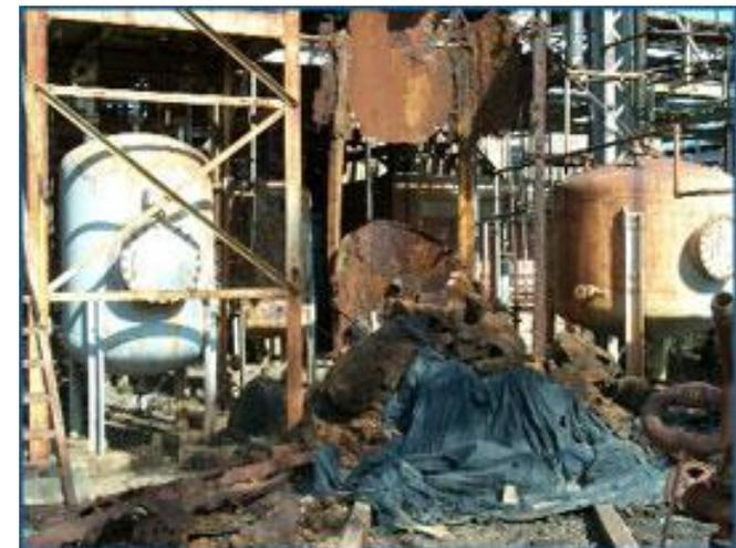
Piles of Sevin, a pesticide, lie rotting at Union Carbide's abandoned plant in Bhopal. Here, the Sevin has corroded through its tank and now festers in the open air.
