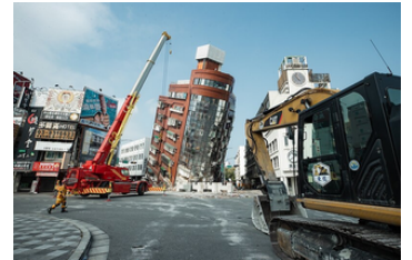
The 'Uranus' building in Hualien City. One of the few buildings to be destroyed from the earthquake. CREDIT: Shufu Liu / Office of the President Flickr
