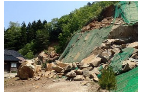
Damage from the earthquake swarm. Source: wikimedia
