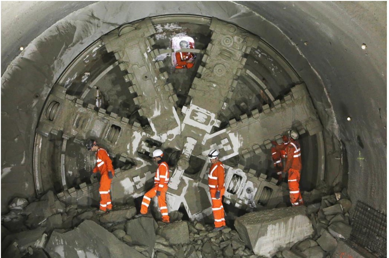
Figure 8 TBM Elizabeth and Victoria arrive at Farringdon © Cross rail
